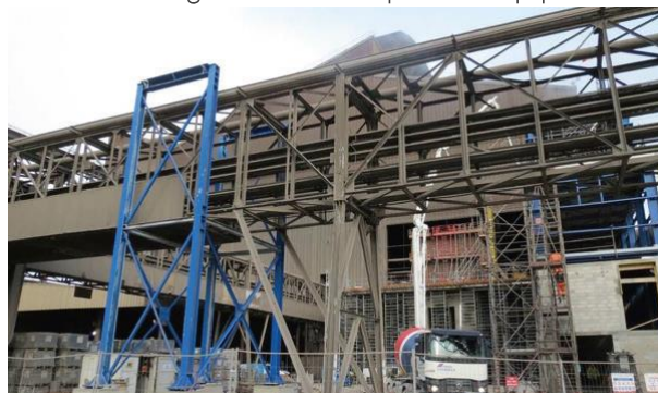
Four poche ArcelorMittal Fos-sur-Mer.
